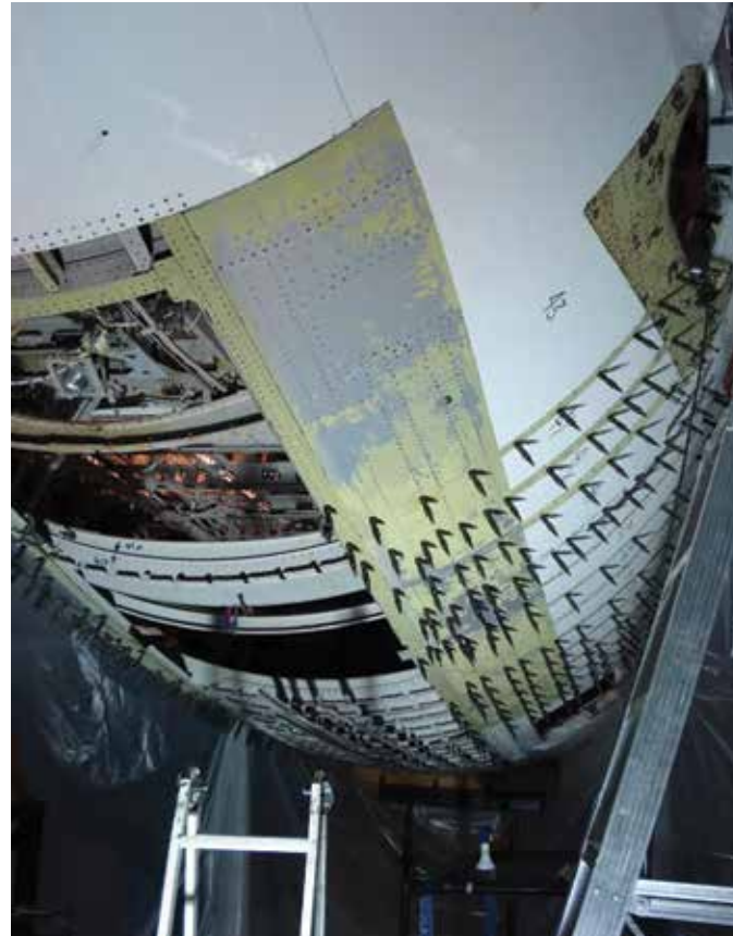
Above: Nine of the fuselage frames had to be replaced.
