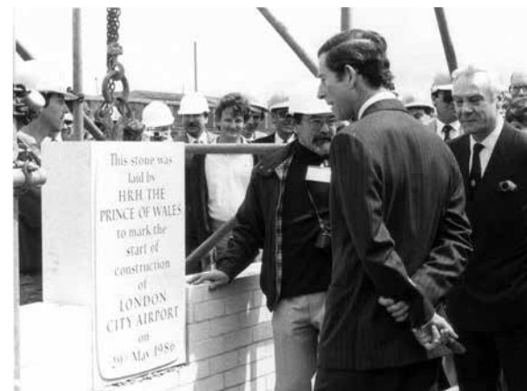
Prince Charles reads the foundation stone plaque.
