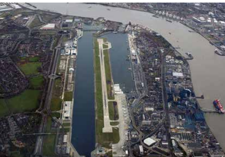
The extended apron is completed.
